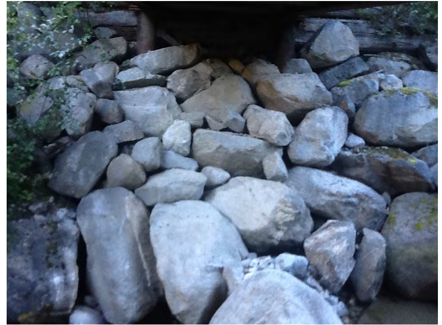
Right Bank Abutment when facing downstream
