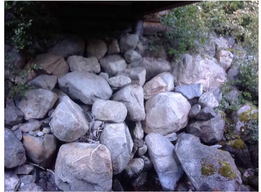
Left Bank Abutment when facing downstream
