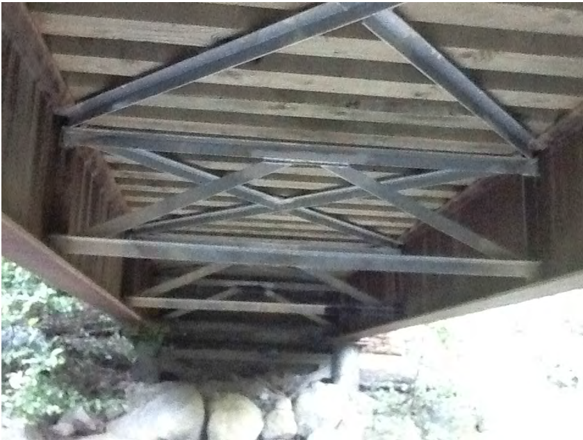
Underside of bridge
