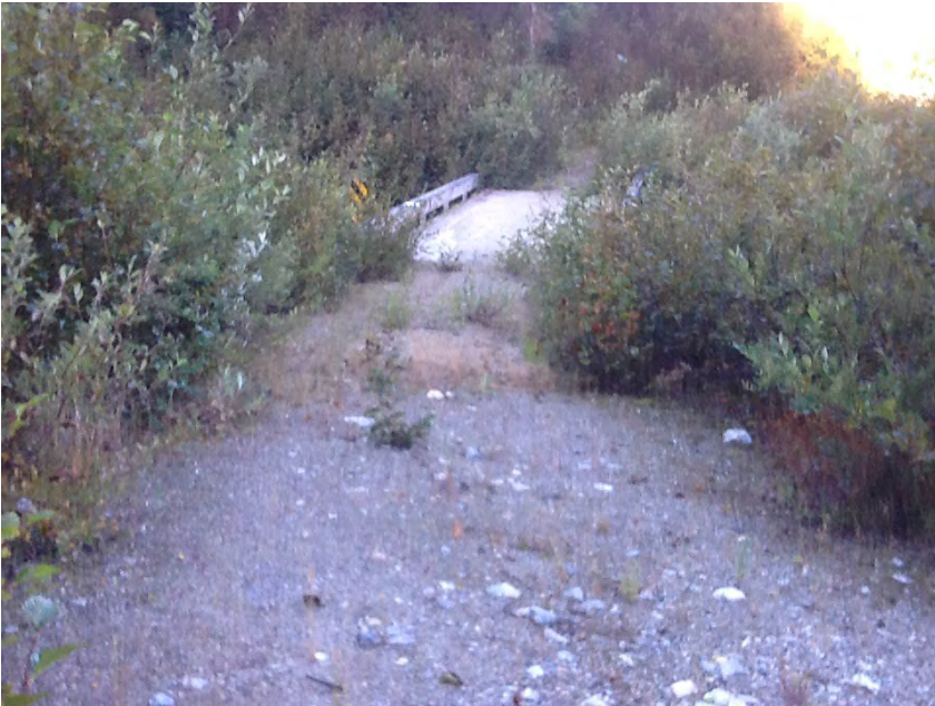
Right approach facing structure
